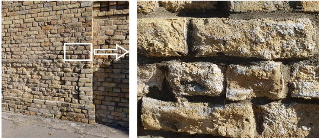
Fig. 1. Moisture destruction of a brick wall in a historic building
