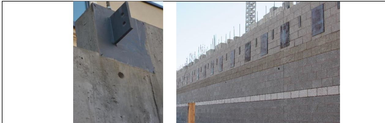
Figure 1. Embeds in concrete and masonry construction.
